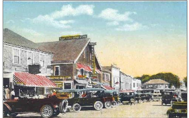
Historic building spacing on the east end of Main Street.
