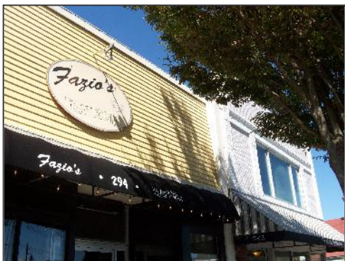
Traditional Main Street storefronts with clapboard siding, built around 1900.
